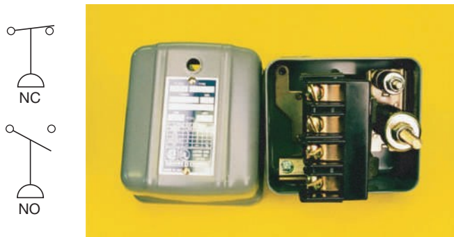
FIGURE 8-4 Line-voltage pressure switch.
