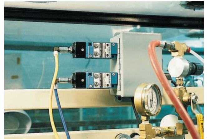
FIGURE 8-11 Pressure-to-current sensor for low pressures.
